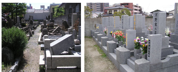
Photo.1 Different overturning ratios of tomb stones showing different strong ground motions during the quake. Just eastern side from the Kego fault showed very high overturning ratio of 20 through 30 % (the left), although the western side from the fault showed only a few percent (the right).
