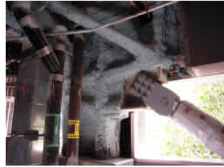
Beam-to-column Connection in the Moment-frame
