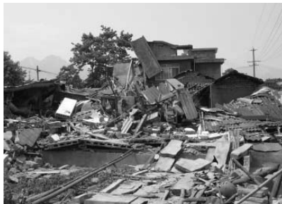
Figure 23. Collapsed residential units
