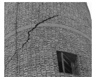
Figure 29. Shear crack in URM water tower
