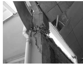
Figure 10. Column flexural failure
