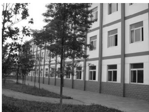
(Grade 0) No damage
