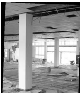
Figure 19. Damaged suspended ceiling
