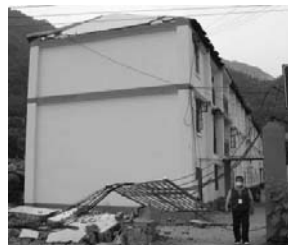
Figure 21. Damaged roof of the building
