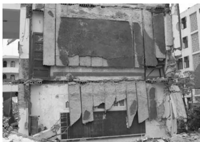
Figure 5. Collapsed floor planks
