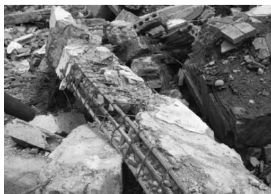
Figure 6. Collapse URM wall and concrete beam
