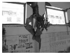
Figure 9. Captive column failure
