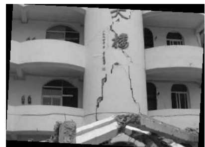
Figure 7. Shear cracks in masonry walls
