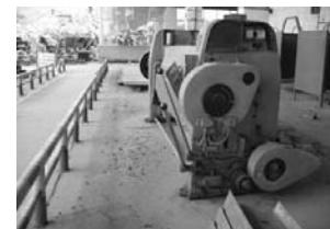
Figure 18. Sliding of un-anchored equipment
