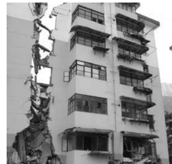
Figure 25. Vertical split and displaced apartment complex
