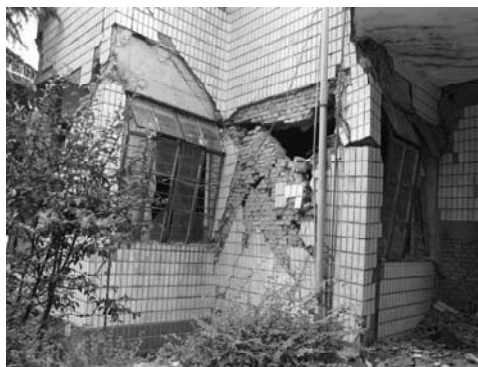
(Grade 5) Collapse or near collapse
