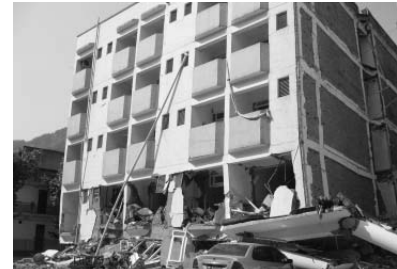
Figure 14. Soft story collapse
