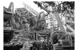
Figure 22. Collapsed Bank of China branch
