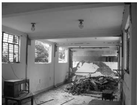
(Grade 4) Severe damage
