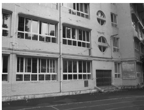
(Grade 3) Moderate damage
