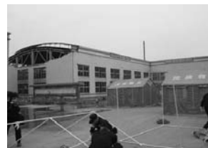
Figure 17. damaged URM wall and emergency tents
