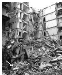
Figure 20. Collapsed corner of the building
