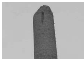
Figure 15. Damaged URM stack
