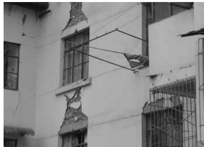
Figure 24. Cracked URM walls
