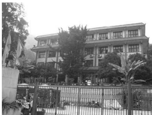
(Grade 1) Slight damage
