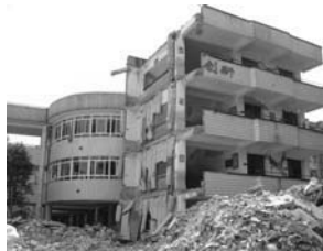
Figure 8. Collapsed primary school
