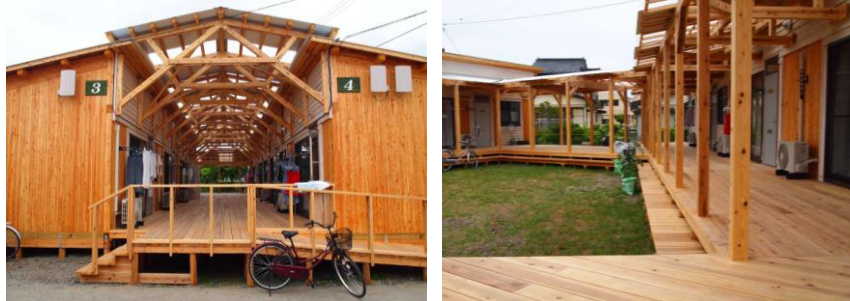
Photo 2: Temporary housing complex at Tono, Iwate Prefecture, comprises two rows of homes with entrances facing across a wooden deck; connecting arcades at right.
