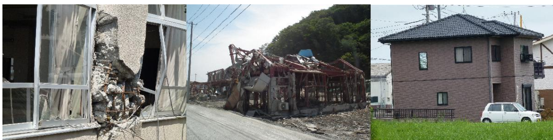
Photo 4: Damage to reinforced-concrete school facility
