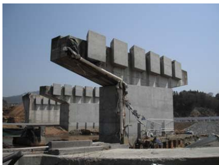
Photo 5: Unseating prevention systems in Numata Bridge nearly intact
