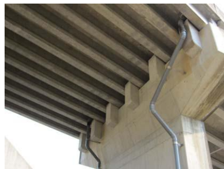
Photo 2: Main girders interconnected and piers reinforced by wrapping method
