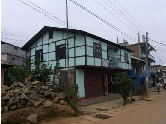
Fig. 3.27. No cracks in the building constructed using “*Centibera*”.
