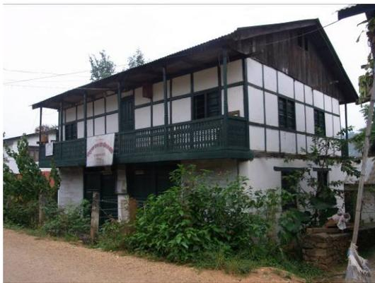
Fig. 3.29. No cracks in the building constructed using *Centibera*.
