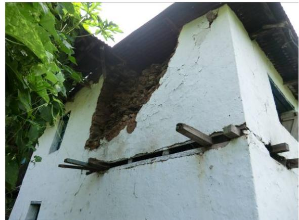
Fig. 3.8. A damaged stone masonry (mud mortar) building: (a) with collapsed wall at the front portion and (b) with collapsed wall at the back portion.
