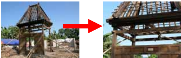
Photo B. 6-7: An old wood structure with `Takik` structure is the only standing structure remains in the whole Pleret village.
