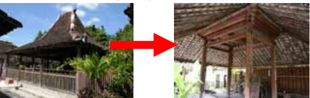
Photo C. 7-8: An old House in `Kota Gede (Old Town), with `Saka Guru` structure stands more than 50 years.
