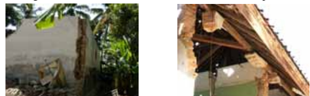
Photo B.2 (left) and B.3 (right): Un-reinforced Brick House with no RC columns between the walls is completely collapsed and the brick wall with no beam is directly connected to the roof system.
