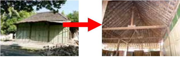
Photo B. 4-5: An old house with wood roof system and lightweight wall still exists while the brick wall additions were collapsed.
