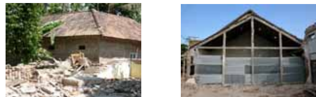
Photo. B.1 (left) and C.5 (right): Houses in Patalan and Kota Gede with rigid RC frame structure remained while others collapsed.
