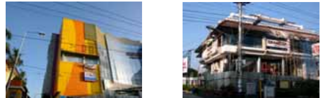
Photo. C.3 (left) & C.4 (right): Saphir Mall and Gramedia Bookstore, private owned shopping mall, damages on glass walls.
