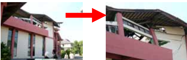
Photo. C.1-2: Among Progo Sport Center damaged in the roof system and cantilever reinforced column on the top floor.
