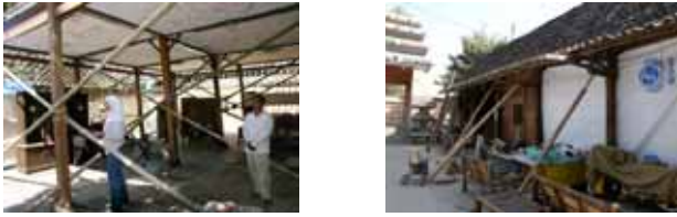
Photo A. 3 (left) and C. 6 (right): Old houses with wood structures, occupants maintain its old wooden structures with temporary bamboos support for undergoing renovation.
