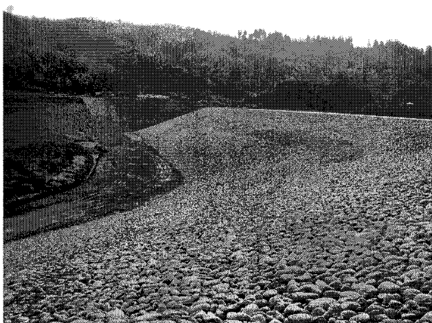
(c) Left Ban-side after Restoration for which Fine Deposits were Removed.
