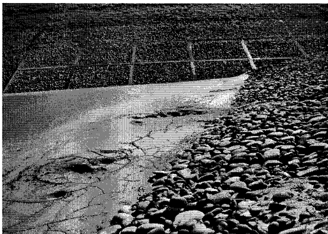
(a) Boiled Sand indicating Liquefaction on the Left Upstream-side.
