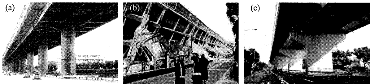
Photo 3 Highway structure collapsed during the 1995 Kobe earthquake. Photo before the earthquake (a), Just after the earthquake (b), and after 18 months from the earthquake (c).
