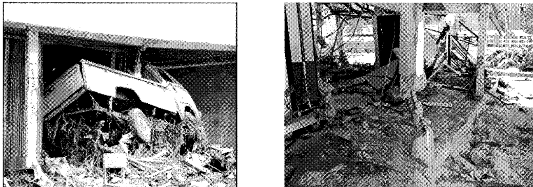
Figure1. Damage due to Impact of Waterborne Massive Objects of the Tsunami caused by the Sumatra-Andaman Earthquake of December 26, 2004 (Ghobarah et al. 2006).
