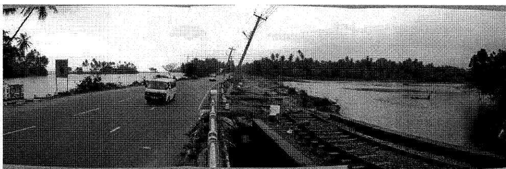
Fig. 7. North Ambalangoda: Electric poles lean to the right, rail tracks had been damaged.
