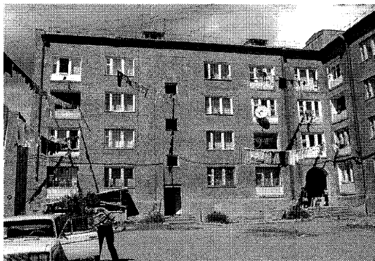
Photo.5 Typical infilled RC frame structure for residence in Ani district, new town in Gyumri.
