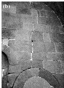
Photo.21(a-d) Hripsime Church in detail. A ladder to balcony (a). Wall cracks repaired with white mortar (b). Equipments measuring ambient motions at the base floor (c). Skirting stone blocks as there is no foundation (d).
