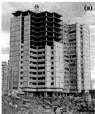
Photo.12(a-c) Tall buildings with lift-slab method are still under construction in Yerevan. There is no wall on the ground level, and outer walls in upper floors are non-seismic.
