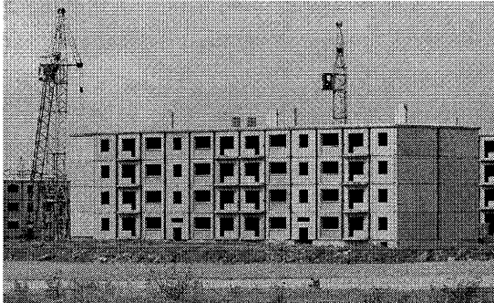
Photo.3 Large panel structure under construction, but nobody is found around the site. (outer Gyumri)
