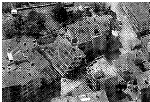
Figure 2 The Terveler building (left) and its “back-to-back” neighbouring building (right), both of which toppled in the earthquake, in opposite directions
