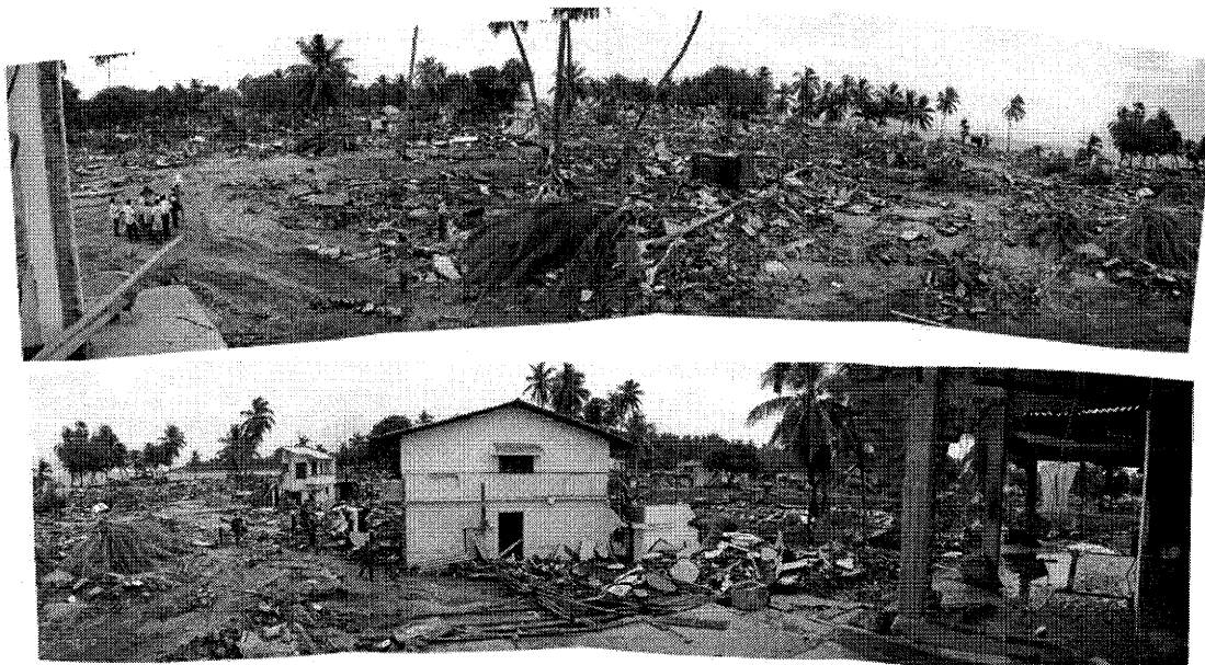
Fig.14. Hambantota: Masonry houses located within a few hundred meters from the coast were completely destroyed, a few more recently constructed houses had less damage.
