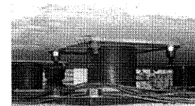
Figure 7 Elastomeric bearing pad.
