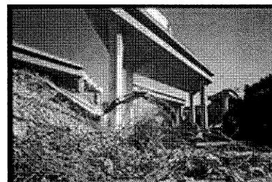
Figure 3 Bridge collapse at in-span hinge
