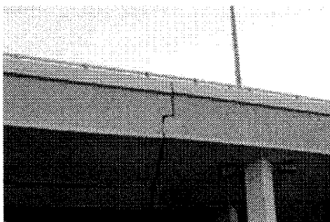
Figure 2 In-span hinge of multi-frame bridge
