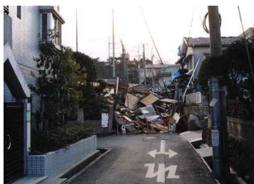
Photo.4 Such condition even after a couple of months (Uozaki, Kobe)
