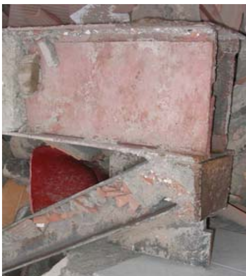
Figure 12 Steel Structures with inappropriate welding that led to the separation of the beam or bracing from the columns.
