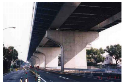
Photo.15 Restored Hanshin Highway after 20 months (Fukae, Kobe)
