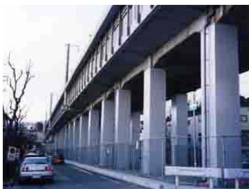
Photo.13 JR-Shinkansen after temporary repairs (Nishinomiya)
