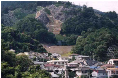
Photo.10 Land failures protected after two years (Sumiyoshi-Yamate, Kobe)
