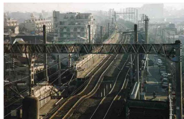
Photo.5 Failure of JR-Super Express called Shinkansen (Nishinomiya)
