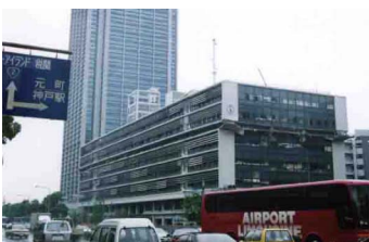
Photo.17 Kobe municipal office just after the earthquake
