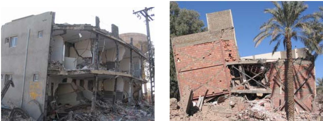
Figure 14 Minimum attention to the country's seismic code, or proper construction techniques, could have prevented many buildings from total collapse.
