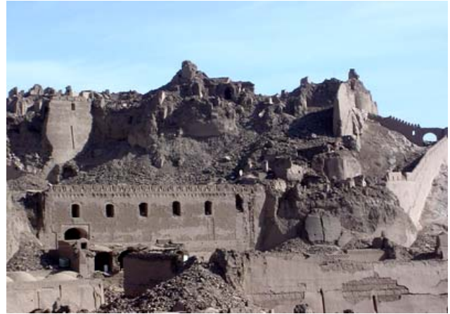
Figure 2 The Arg-e Bam after earthquake.
