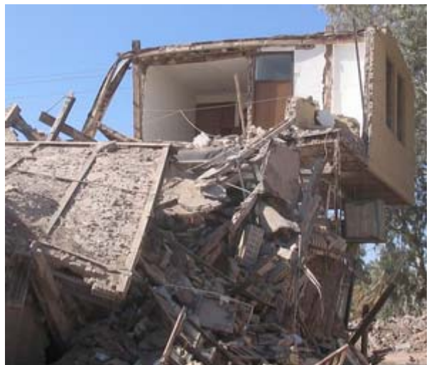
Figure 10 collapsed un-reinforced masonry buildings with steel jack arch type roofs.
