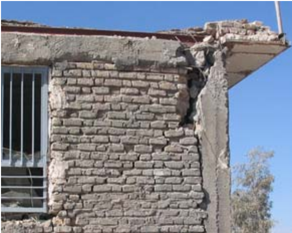
Figure 11 The reinforced masonry buildings with seperated vertical bonding beams, inappropriate connection detailing and poor concrete quality.
