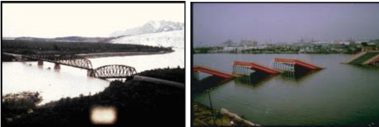
Figure 1: Failure of bridges in earthquakes; (a): Million Dollar Bridge after the 1964 Alaska earthquake; (b): Showa Bridge after the 1964 Niigata earthquake. Photo courtesy NISEE.
