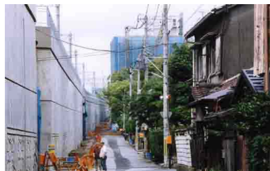
Photo.14 Restored railway (left) and old houses alive (right) (Okamoto, Kobe)
