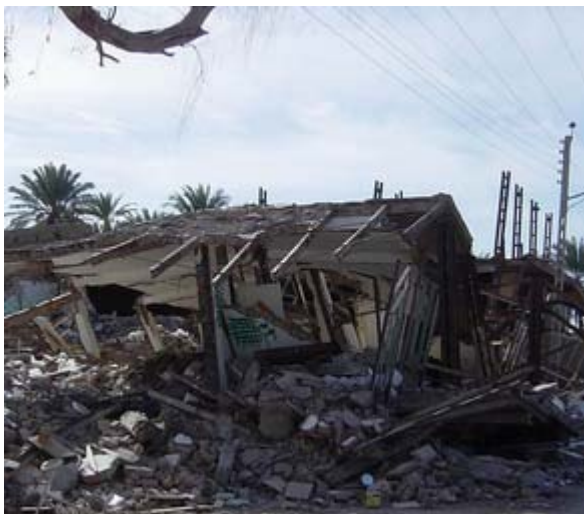
Figure 10 collapsed un-reinforced masonry buildings with steel jack arch type roofs.
