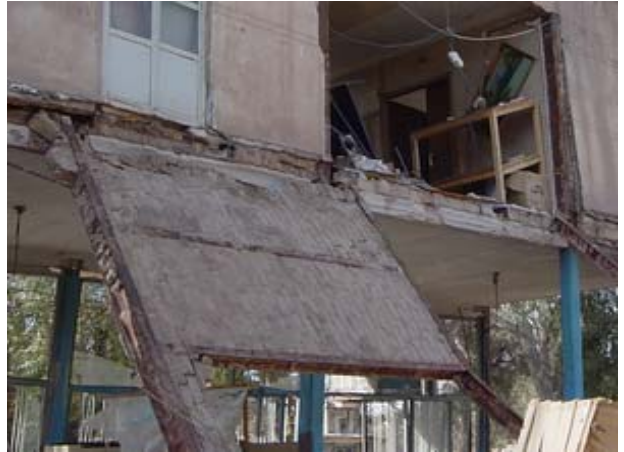
Figure 9 The un-reinforced masonry buildings and an example of steel jack arch type roofs.
