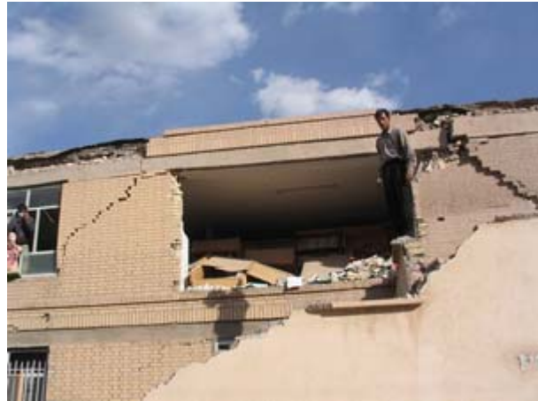
Figure 11 The reinforced masonry buildings with seperated vertical bonding beams, inappropriate connection detailing and poor concrete quality.
