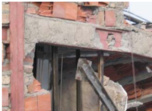
Figure 12 Steel Structures with inappropriate welding that led to the separation of the beam or bracing from the columns.
