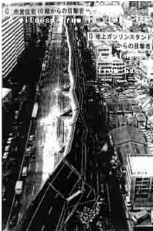
Photo.19 Overturning failure of Hanshin Highway and the location of watchers
