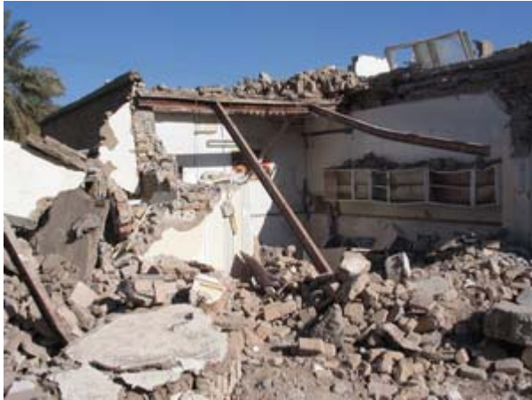
Figure 9 The un-reinforced masonry buildings and an example of steel jack arch type roofs.
