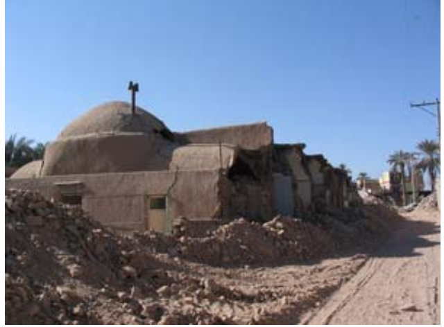
Figure 8 The adobe buildings with dome or arched type roofs.
