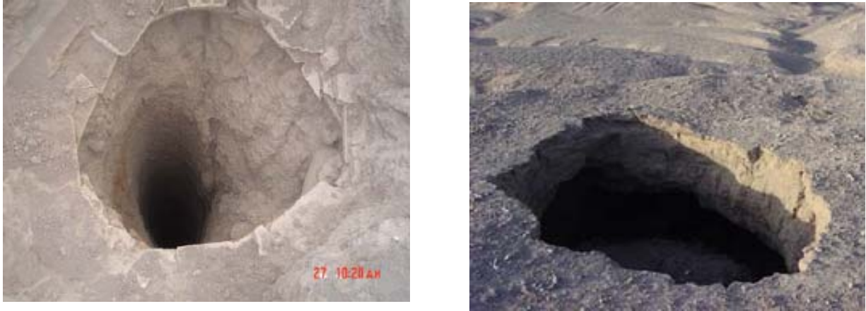
Figure 21 A view of the opening of vertical shafts of the qanats and their type of failure caused by the Earthquake[6].
