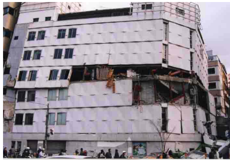
Photo.8 Walking people did not care about collapsed buildings (Motomachi, Kobe)
