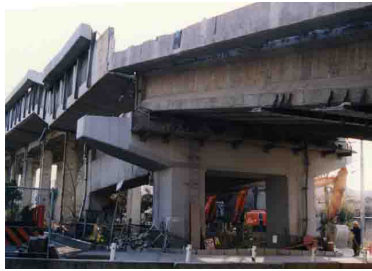
Photo.11 JR-Shinkansen with heavy Beams and columns (Nishinomiya)
