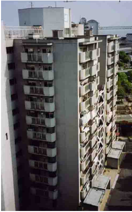
Photo.20 RC-building built with the older building code
