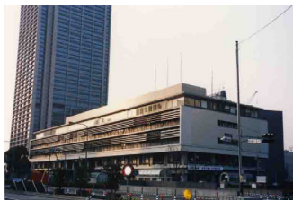
Photo.18 The same building with Photo.17 after a couple of years
