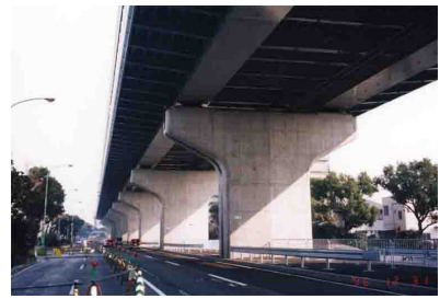
Photo.15 Restored Hanshin Highway after 20 months (Fukae, Kobe)
