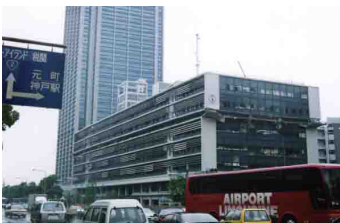
Photo.17 Kobe municipal office just after the earthquake
