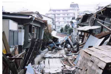
Photo.2 Collapsed houses disturbed rescue activities (Uozaki, Kobe)
