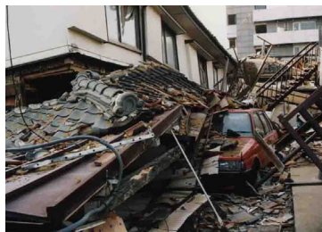
Photo.1 Typical example of collapsed wooden houses (Nishinomiya)
